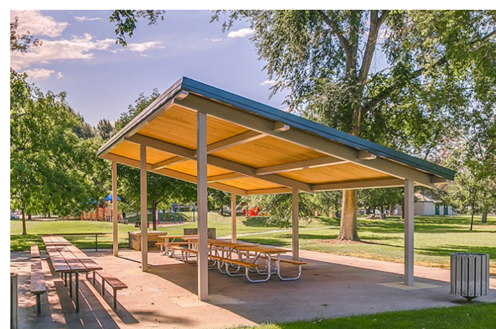
WEATHER PROTECTIVE CANOPY
