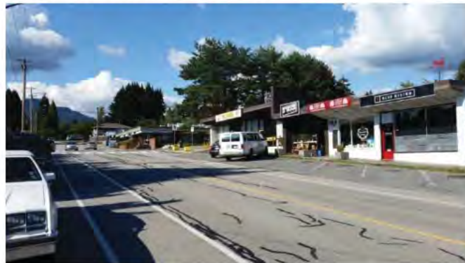
Figure 19 - Queensbury Ave. (left) street view
