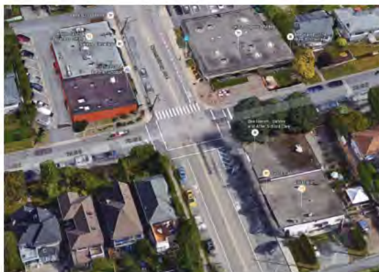
Figure 15 - Queensbury Ave. (left) overhead view
