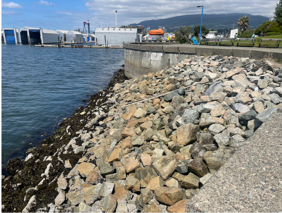
Figure 11: A Picture of the rocks that support the seawall shows the gradual decline towards the water surface.
