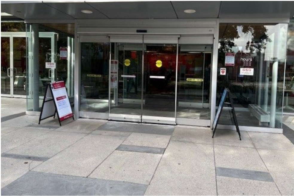
Entrance way to the building showing large accessible automatic doors.
