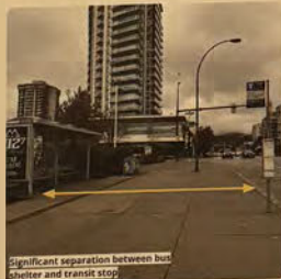
Significant separation between bus shelter and transit stop.
